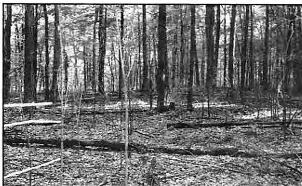
Prior to a shelterwood seed cut, herbicide was used to kill understory trees and remove low shade. The purpose of the site preparation was to allow oak to establish under the high shade of the overstory. Photo by Dave Feicht, USDA Forest Service Morgantown, West Virginia
