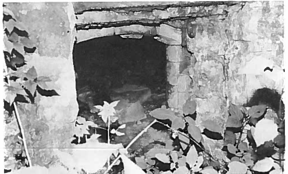
Although vegetation is rapidly hiding the coke ovens at the town of Sewell, many of the nearly 200 beehive-shaped coke ovens remain intact and visitors can see first hand how coke was produced in this thriving community over 100 years ago.
