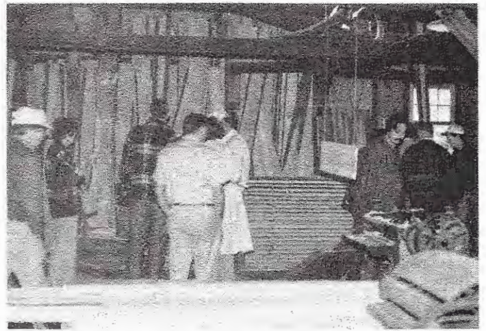
Restored Sawmill at Double Trouble
