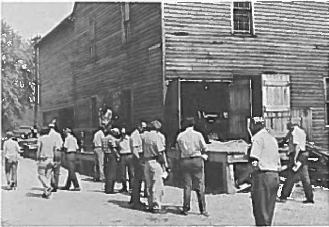
The rebuilt water-powered sawmill at Basto State Park was given the once-over from top to bottom by many on the summer meeting tour. Several walked out with souvenir cedar shingles.
