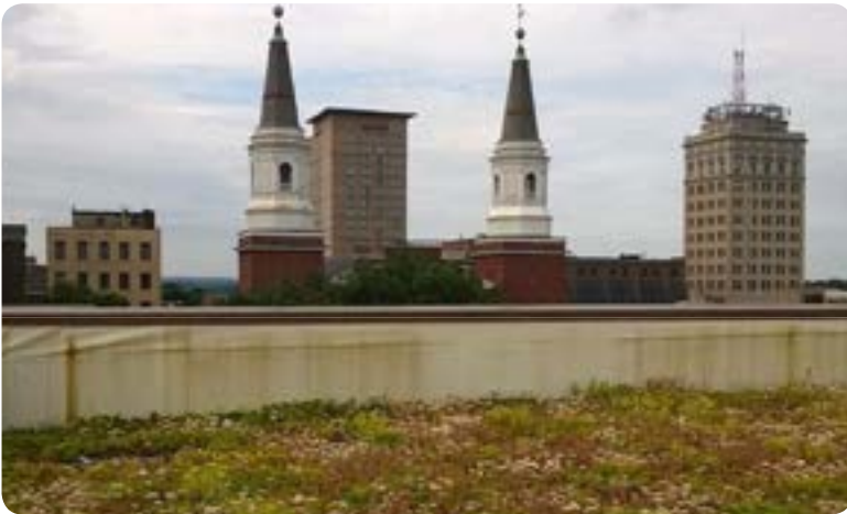
LEED Silver City Hall Annex green roof in its second year.
