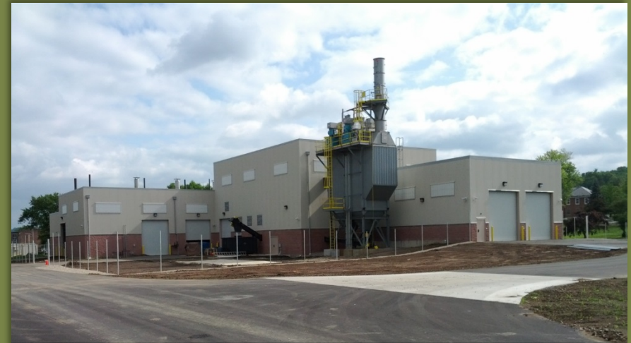
Example Project: 1 million ft 2 VA Hospital Campus Chillicothe, OH Biomass CHP System Heating/Cooling
